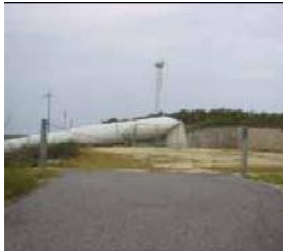
Wind turbine No. 3
