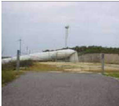
Wind turbine No. 3
