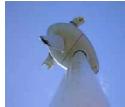
Wind turbine No. 6
