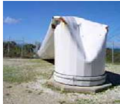
Wind turbine No. 5
