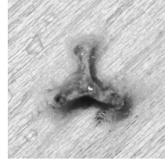
Fig. 2: A tetrapod structure on ceiling, as the basic building block in honeycomb construction.
